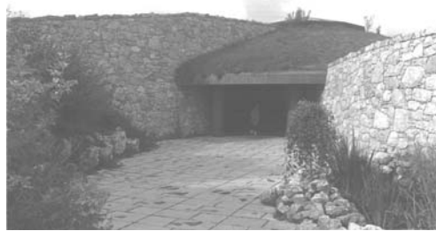
Figure 2.30 The Navan Visitor Centre: the building is buried within a grass-covered mound and is centrally lit with clerestory lighting
